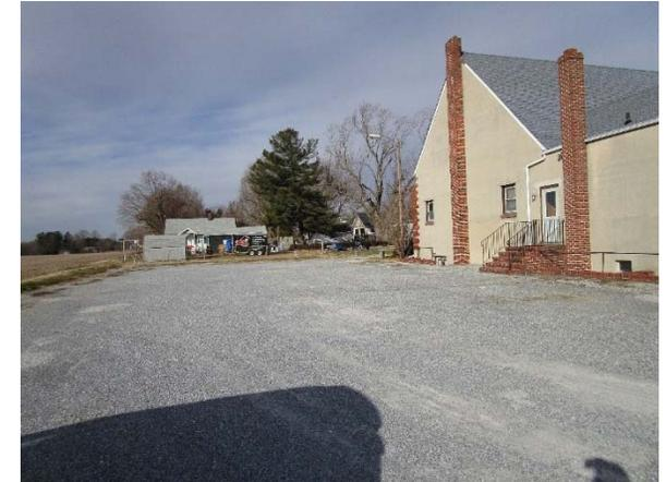
A rain garden can be installed at the northwest corner of the building next to the downspouts. The back half of the parking lot in the back of the building can be replaced with pervious pavement to capture runoff from the rooftop. A preliminary soil assessment suggests that the soils have suitable drainage characteristics for green infrastructure.
