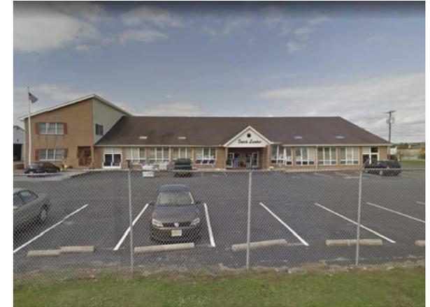
Pervious pavement can be installed in a strip along the south end of the front parking lot to capture a large portion of the parking lot stormwater runoff. A preliminary soil assessment suggests that more soil testing would be required before determining the soil's suitability for green infrastructure.
