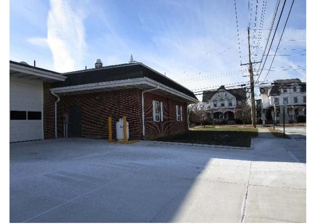
The downspout at the garage door at the north side of the building can be redirected to a cistern. The collected water can be used to wash vehicles or water the existing landscape. A rain garden can be installed at the northwest corner of the building, and the two downspouts in the front of the building can be redirected to the rain garden. A preliminary soil assessment suggests that more soil testing would be required before determining the soil's suitability for green infrastructure.
