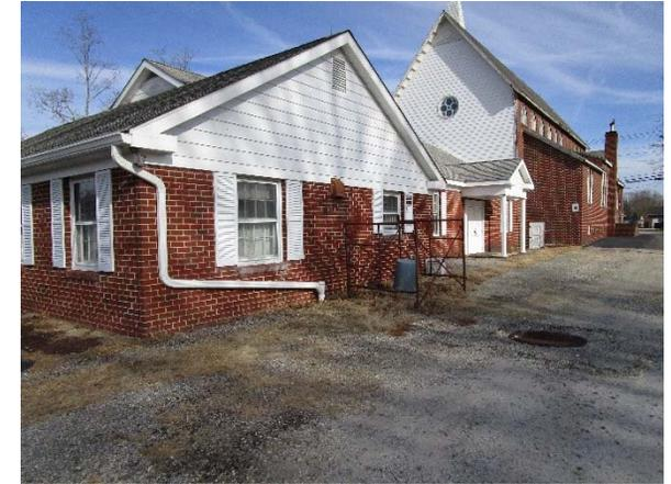
Planter boxes can be installed at the southwest and southeast corners of the building. Approximately four and two planter boxes, respectively, would be connected together to receive runoff from each downspout. These are wooden boxes that provide an opportunity to beneficially reuse rooftop runoff while removing pollutants. A preliminary soil assessment suggests that more soil testing would be required before determining the soil's suitability for green infrastructure.
