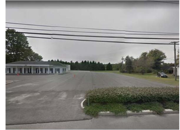
Pervious pavement can be installed in a strip along the west side of the parking lot to the west of the building to capture a large portion of the parking lot's runoff. A rain garden can be installed at the southwest corner of the parking lot in the turfgrass area to capture, treat, and infiltrate stormwater runoff from the parking lot as well. A preliminary soil assessment suggests that the soils have suitable drainage characteristics for green infrastructure.
