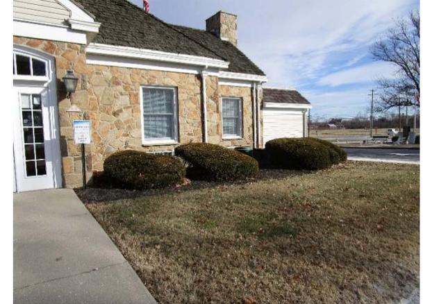
A rain garden can be installed in the front of the building to capture, treat, and infiltrate runoff from the driveway area. The pervious pavement can be installed on the south side of the building to capture runoff from the sidewalk, roof, and parking lot. A preliminary soil assessment suggests that more soil testing would be required before determining the soil's suitability for green infrastructure.
